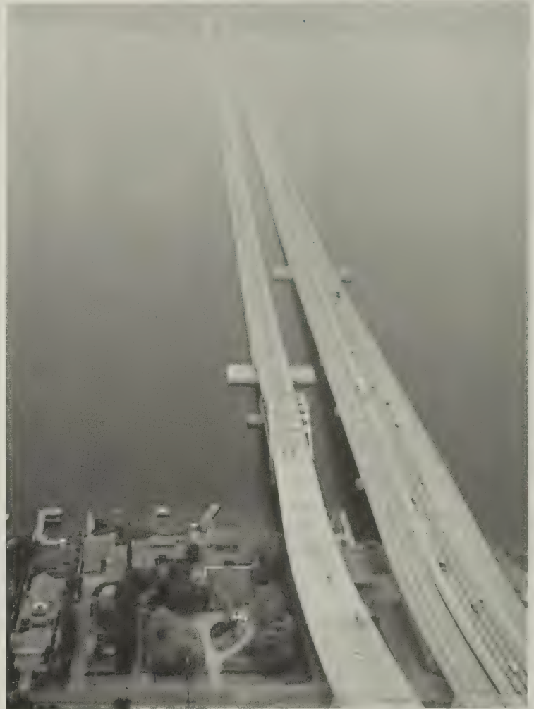
The Lacey V. Murrow Bridge in Washington state was recognized as an outstanding engineering achievement. The new bridge, shown on the left, opened to traffic on September 12, 1993. The floating portion of the bridge is two kilometers (6,600 feet) long.
