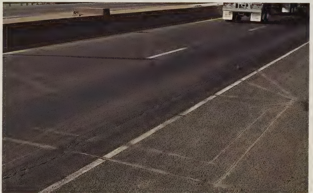
Truck speed can be determined using a pair of embedded inductive loop detectors or piezo sensors.
