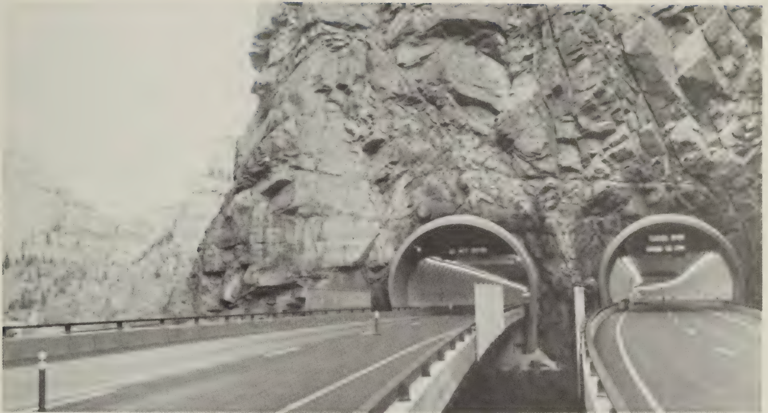
Hanging Lake Tunnel in Colorado's Glenwood Canyon
