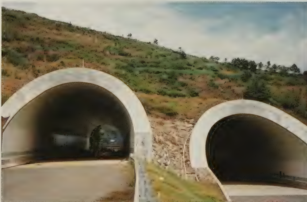
The Hospital Rock "cut and cover" tunnels.
