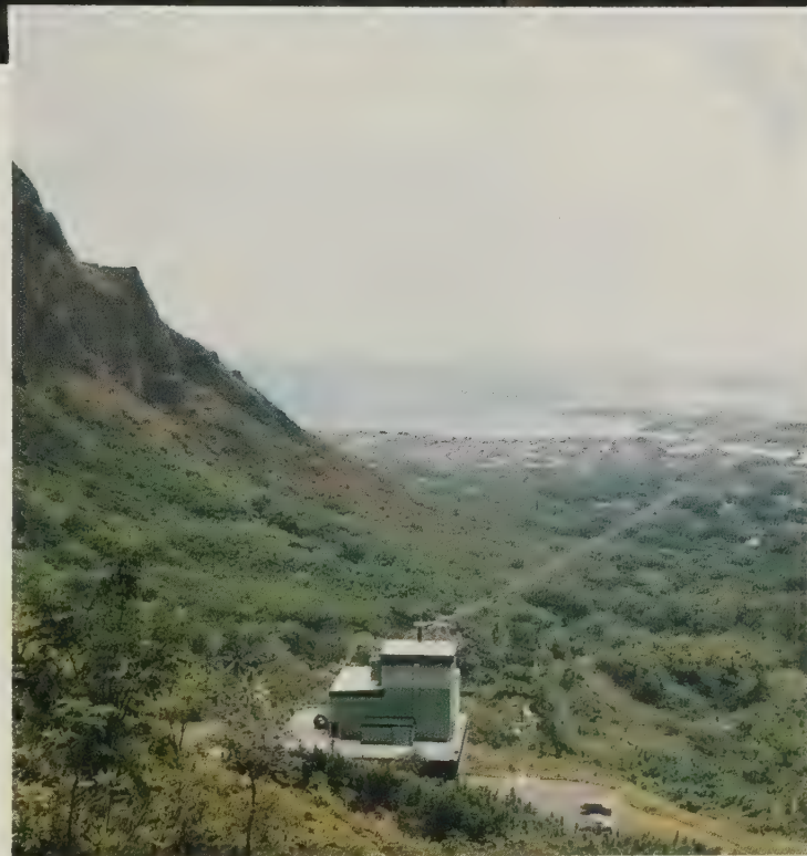
Right. The Coast Guard Omega Station located on the windward side of the Koolaus near the mouth of the Trans-Koolau Tunnels. This station causes large, insulated objects nearby to become charged, posing the threat of shocks to workers and users of H-3. Several countermeasures have been taken to eliminate this problem.
