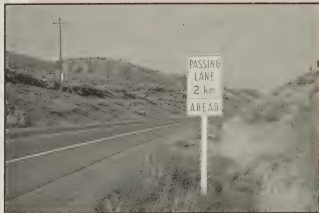
Signs, in addition to pavement markings, are helpful.
