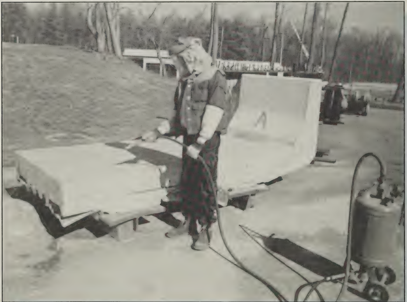
Figure 1.—Concrete deck section under sandblast.
