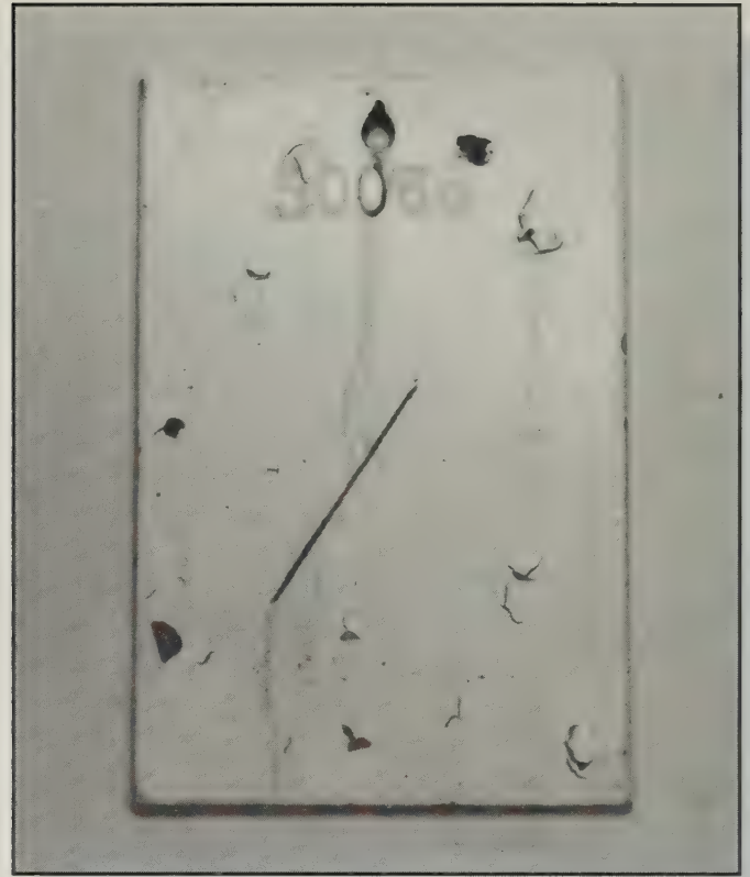
Figure 2.—Condition of the low-VOC epoxy mastic/acrylic epoxy after 3,000 hours of cyclic salt-fog/freeze exposure.
