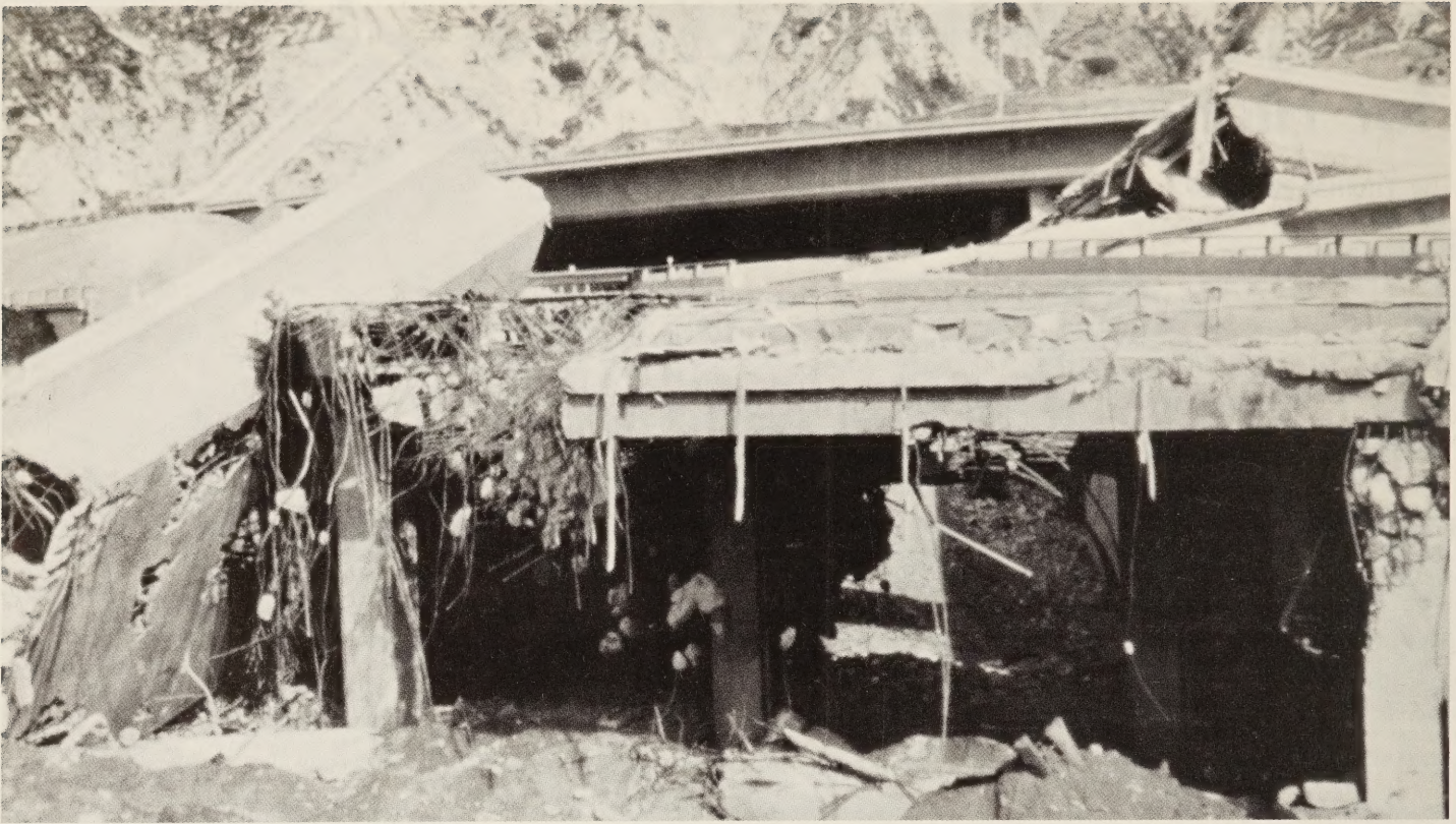
Figure 1.—Damaged bridge, Golden State Freeway, San Fernando Earthquake, 1971.
