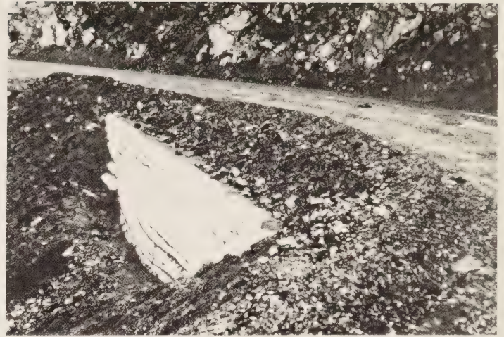
Figure 6. — Fabric-reinforced soil wall.
