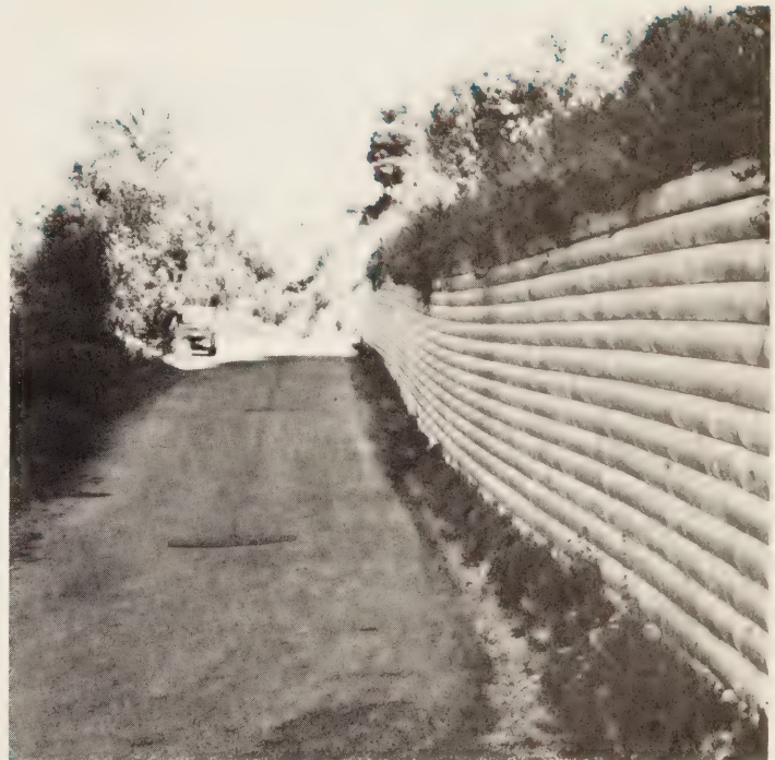
Figure 4. — First highway use of modern Reinforced Earth wall, near Nice, France.
