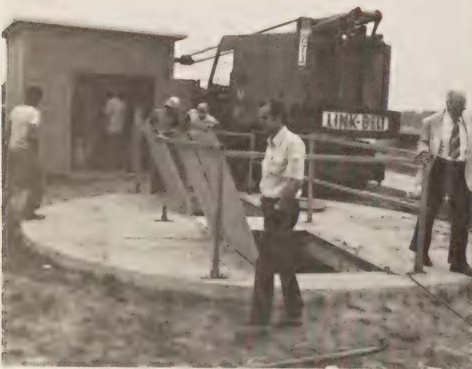
Figure 5.—Caisson for submersible pumps.
