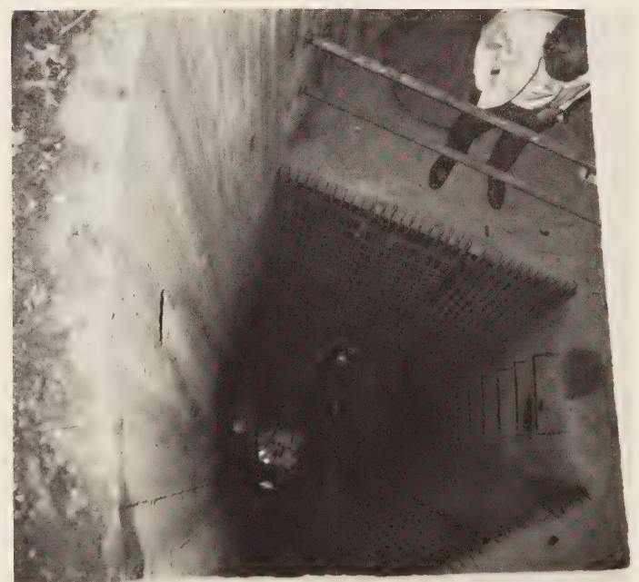
Figure 3.—Caisson-type wet-pit station.
