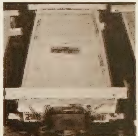
Figure 20.—Slab 210: Epoxy coated with holidays, 0.24 percent bare area, top mat only, 8.7 kg CF/m 3 (14.7 lb CF/yd 3 ), April 1982.
