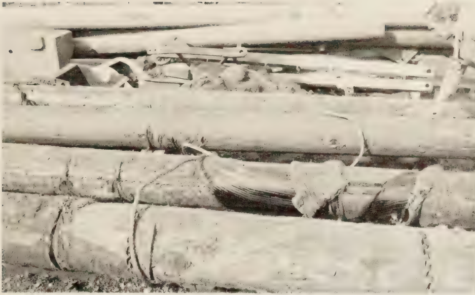
Figure 9.—Extracted test piles showing localized cable-damaged coating.
