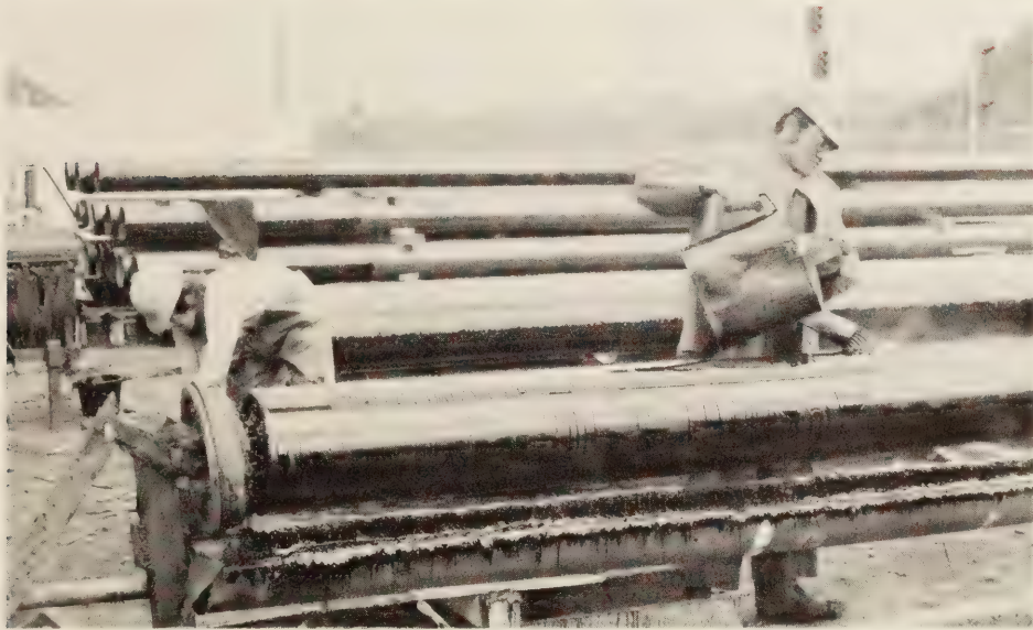
Figure 10.—Production piles in lathe receiving bitumen coating.
