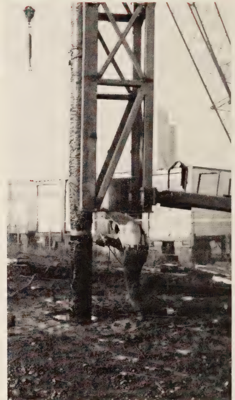
Figure 8.—Splicing test pile No. 1 in leads.
