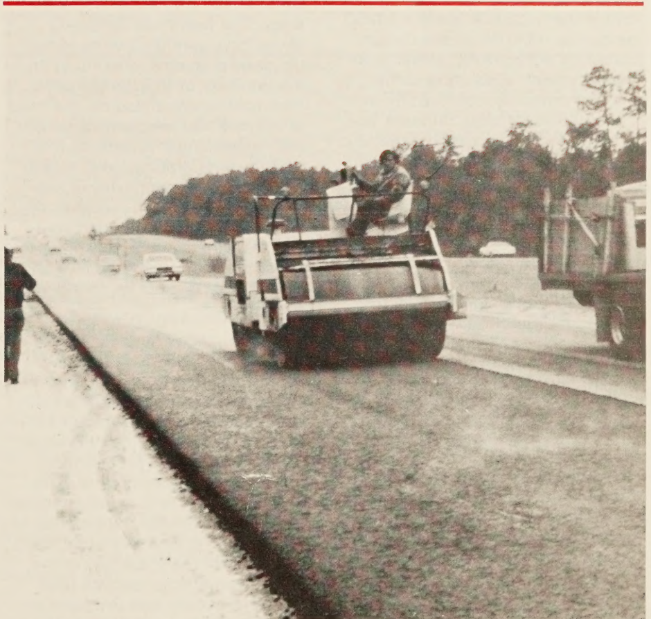
Figure 2.—Compaction of Sulphlex pavement in Florida, 1980.
