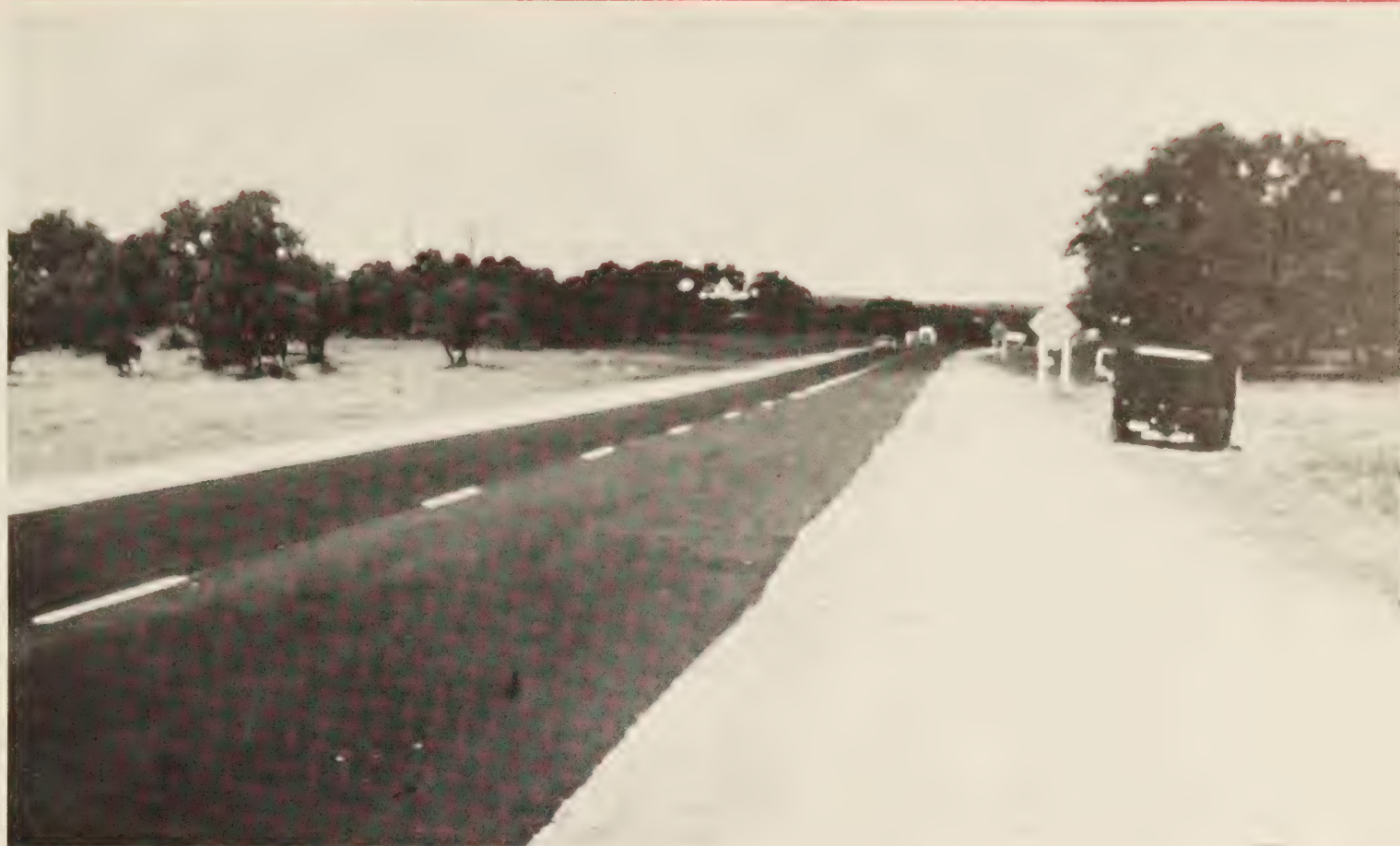
Figure 3.—Sulphlex pavement, Loop 1604, San Antonio, Tex., September 1980.
