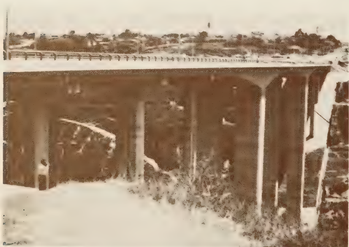
Figure 7.—Undamaged bridge with joint restraining devices provided.
