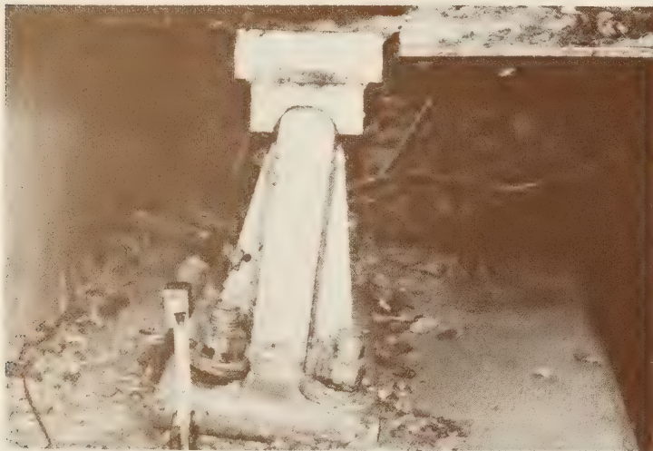
Figure 6.—Tipped bearings.
