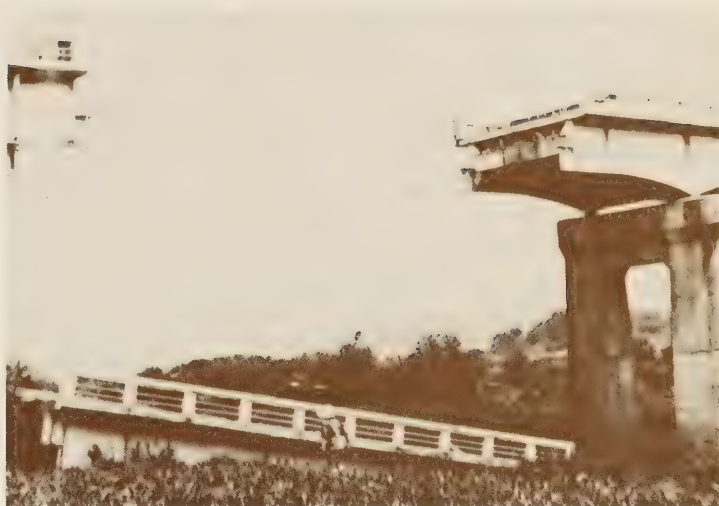
Figure 9.—Collapsed span.
