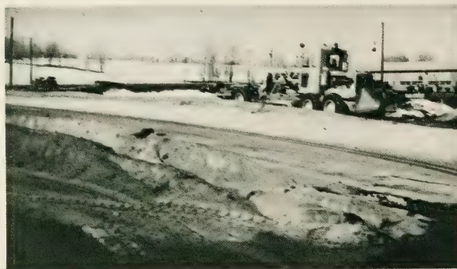
Figure 2.—Sand and salt being mixed with a motor grader.
