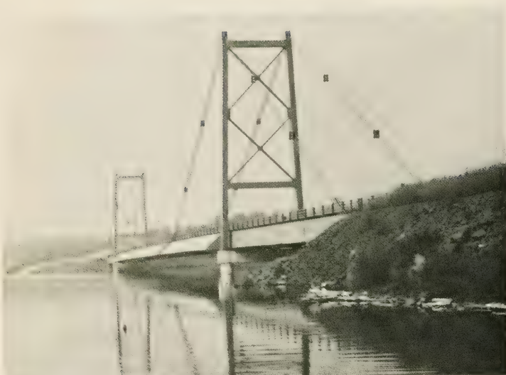
Figure 4.—The modified Long's Creek Bridge.
