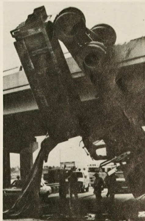
Figure 12.—Straight truck and bridge rail accident.
