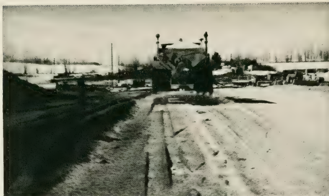
Figure 1.—Spreading salt to be mixed.
