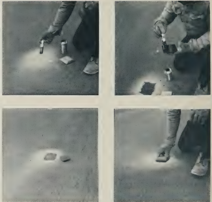
Figure 3.—Installation of pressure-sensitive butyl-backed marker.
