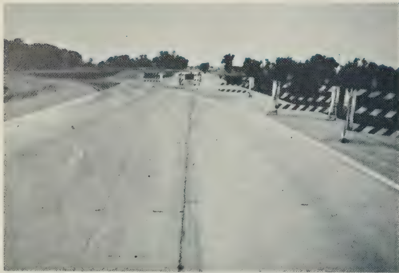
Figure 1.—Daytime view of construction detour.
