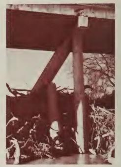
Figure 5.—The lateral forces of water against a large debris accumulation caused the destruction of this bridge pier.
