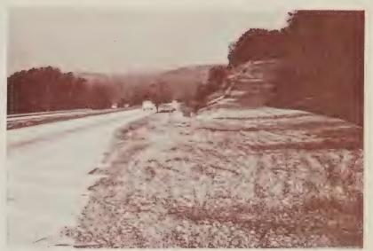
Figure 2. — Arrester bed ramp being constructed.
