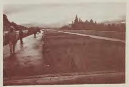
enough. Possibly a larger size aggregate or a different filter material should be used. Sufficient amounts of ponded water, frost, snow, or ice could render the arrester bed ineffective.
