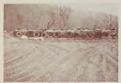
Figure 4. — Arrester bed ramp with attenuator.
