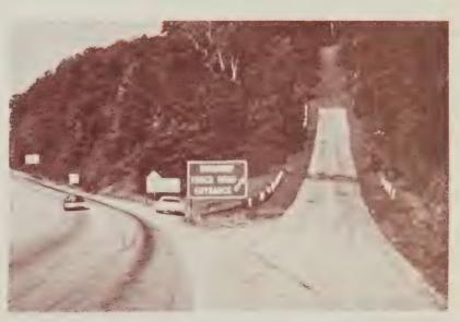
Figure 3.—Combination arrester bed and gravity ramp.
