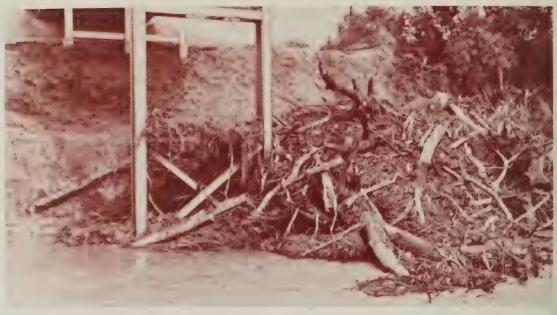
Figure 2.—Massive vegetation debris accumulation on a bridge pier.
