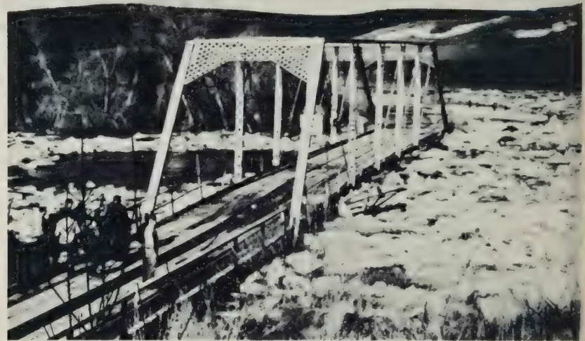
Figure 2.—Ice shoving on bridge at Logan, Mont., 1963. (2)
