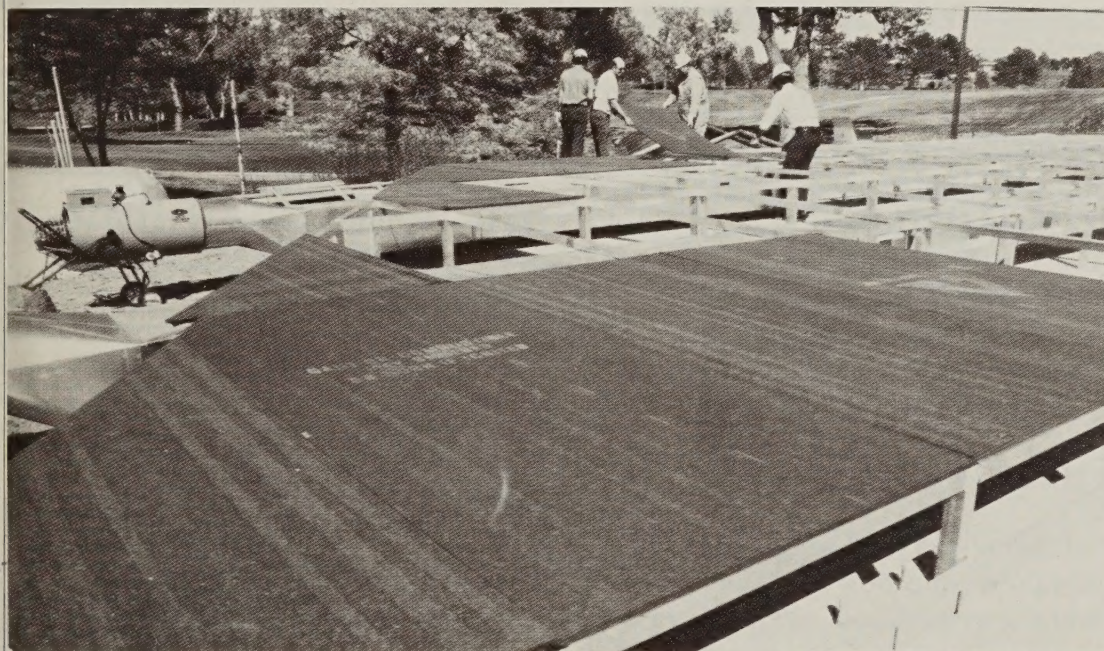
Figure 2.—Fiber building board that formed the insulated top, ends, and sides of the enclosure.
