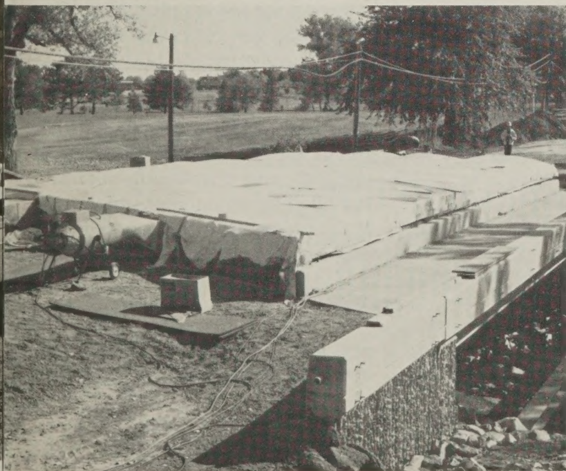
Figure 3.—Completed enclosure in operation on the bridge.
