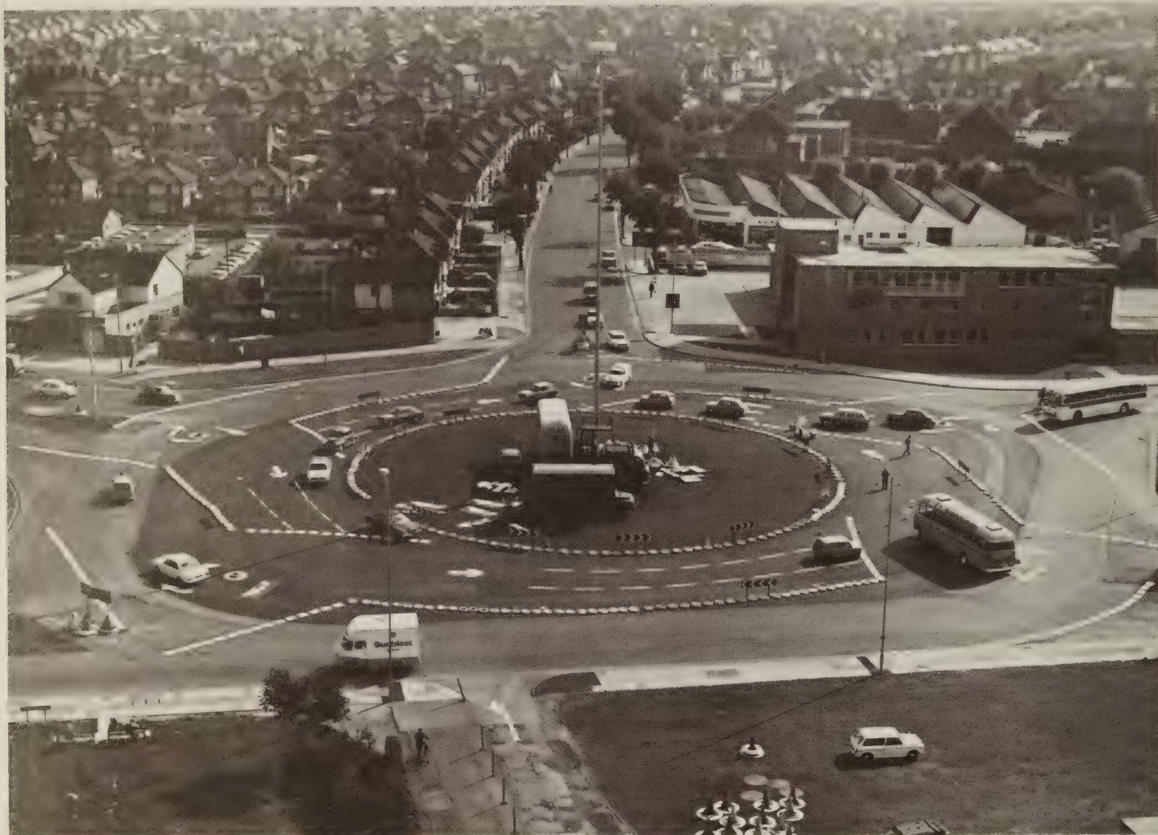
Tests on roundabout intersection design in the United Kingdom.
