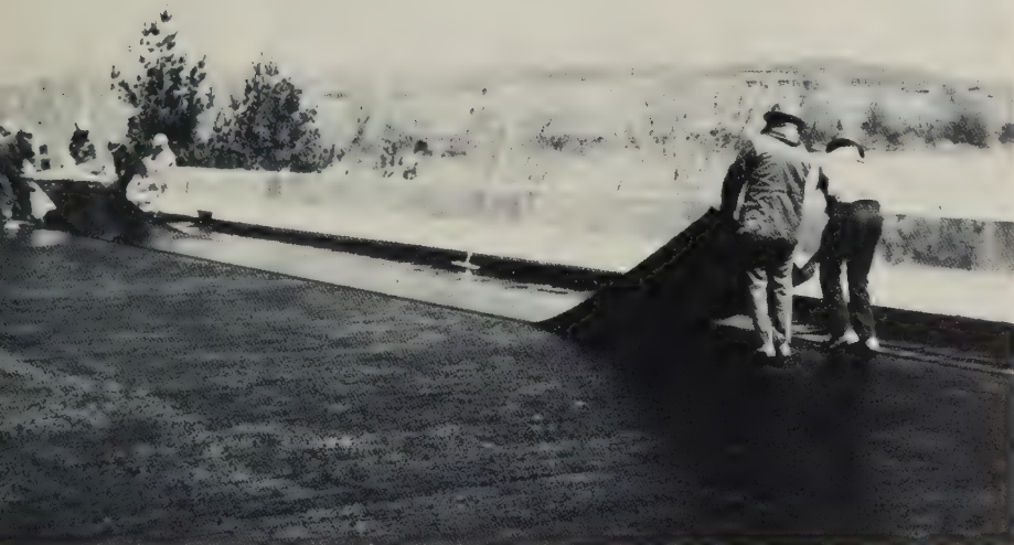
Figure 1.—Applying preformed sheet membrane.
