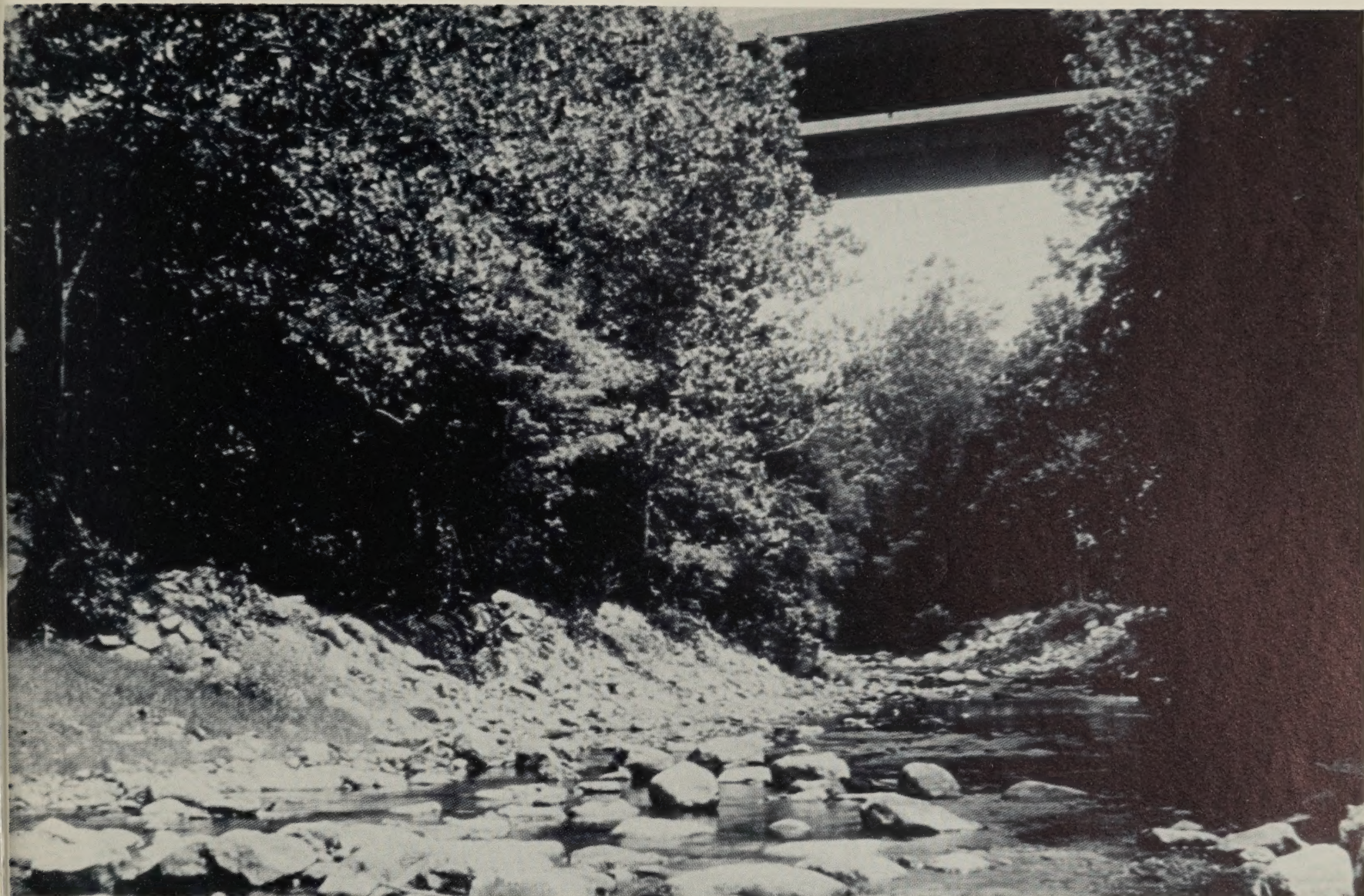
Figure 4.—Single spans protect sensitive aquatic environment.
