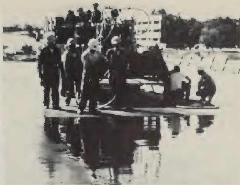
Figure 2.—Applying liquid membrane.
