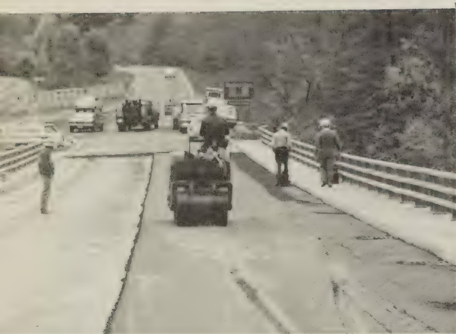
Figure 4.—Placing conductive overlay around anodes on an existing bridge.
