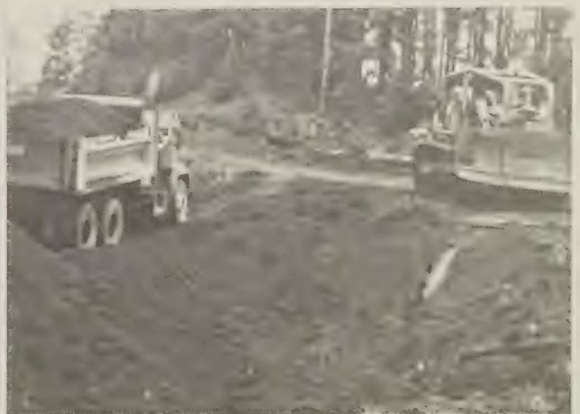
Figure 2.—Sawdust used for emergency repair of this highway.
