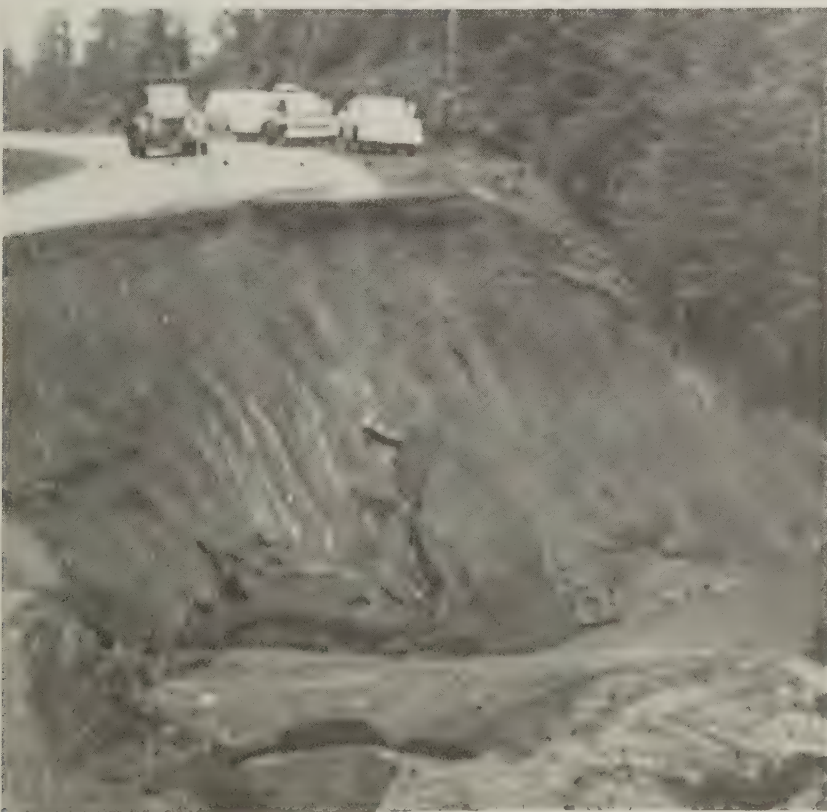
Figure 1.—State Route 101 closed because of major slide—March 1972.
