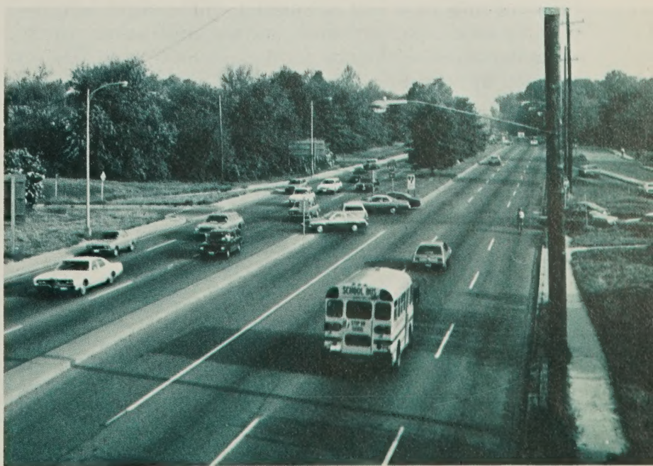
Figure 3.—At unsignalized diamonds in suburban areas with large demands, required driver maneuvers generate numerous conflicts.
