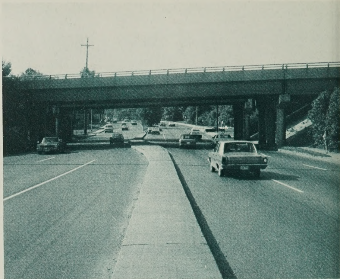
Figure 5.—A separate left-turn lane.
