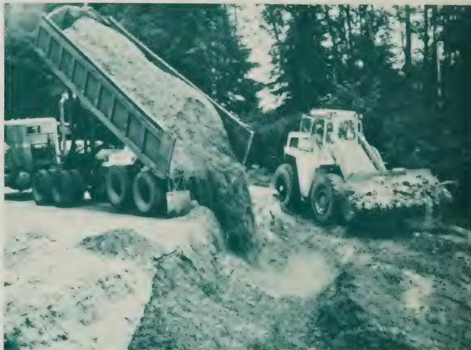
Figure 5.—Sawdust being dumped into the excavated site.
