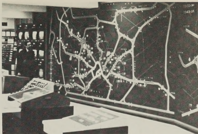
Figure 6.—Map display room at the traffic control center of Metropolitan Expressway Public Corporation, Japan.
