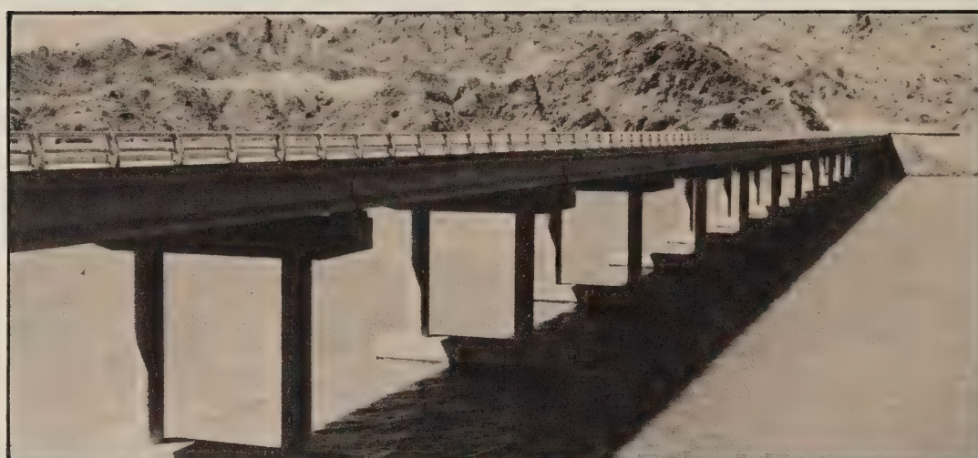
Figure 2.— Analysis and rating of cast-in-place and prestressed concrete bridges are in the system's scope.
