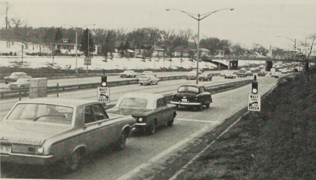
Figure 4. — Chicago ramp signals.
