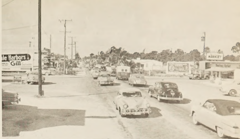
Primary highway of the 1940's—before access control.
