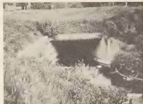
Figure 7.—Side-tapered culvert near Lexington, Va.
