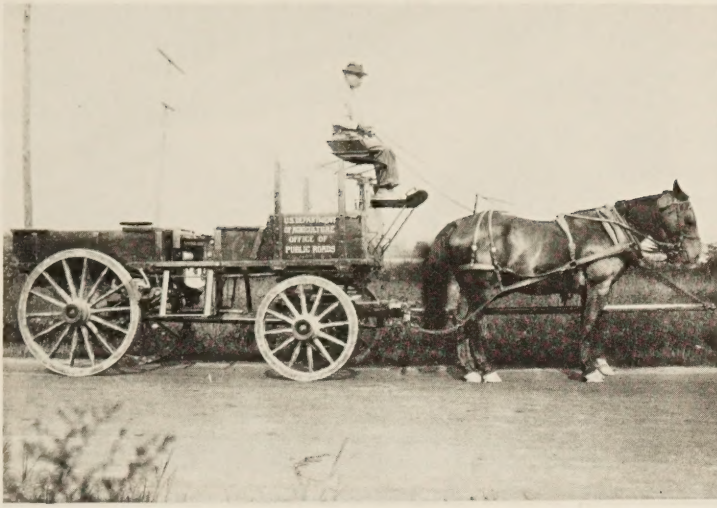
Figure 1.—Early skid measurement system (about 1905).
