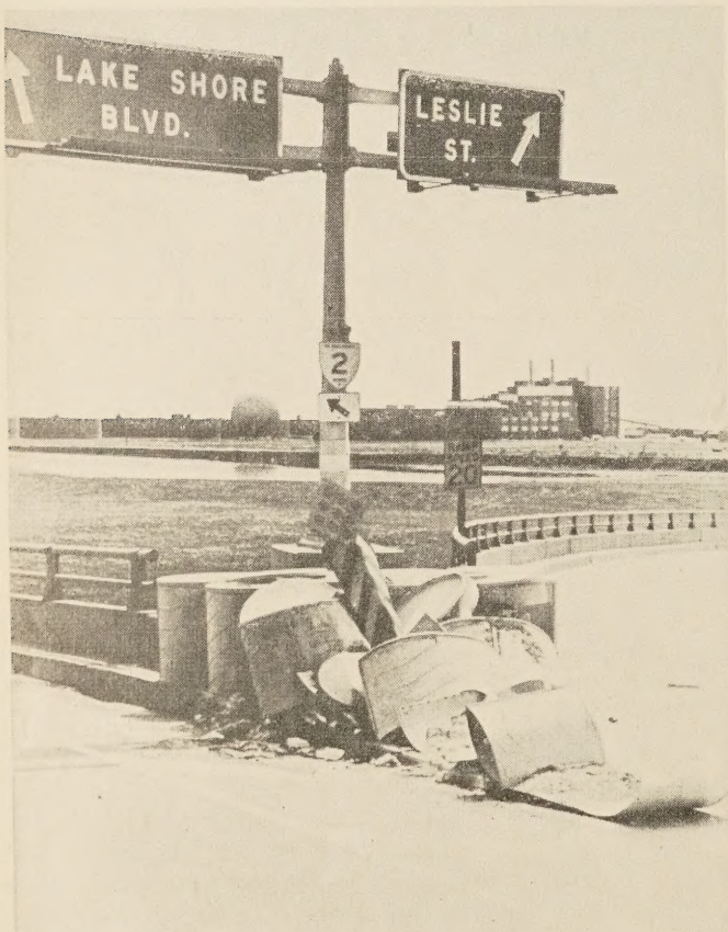
Figure 14.—Typical accident damage to Fitch Inertial barrier.
