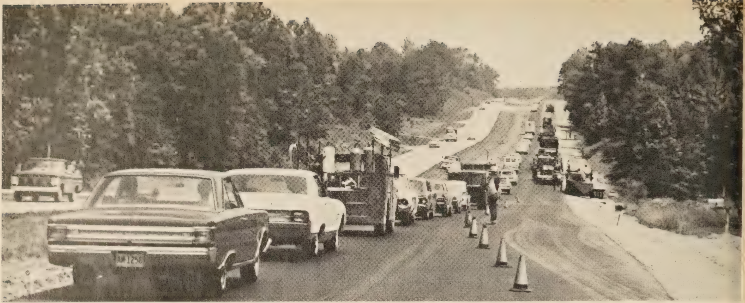
Resurfacing—one method of retiring pavement discussed in this article.
