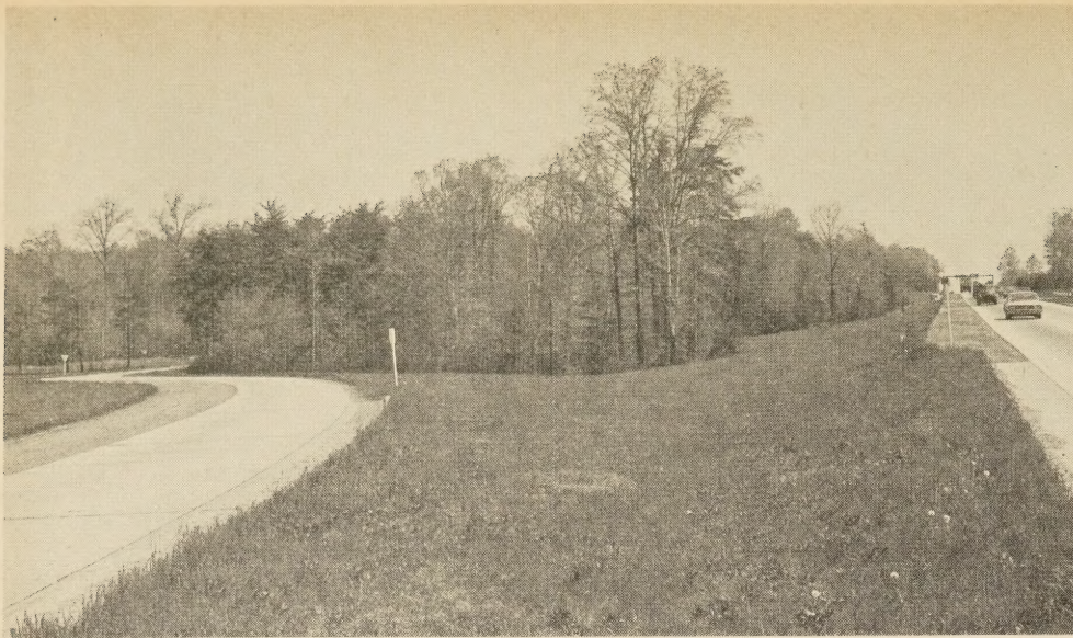
Figure 6.—Dense ground cover of turf and unobstructed sight distances are important aspects of highway safety.
