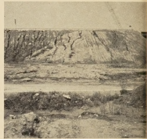
Figure 2.—Erosion control must be considered during design and location deliberations.
