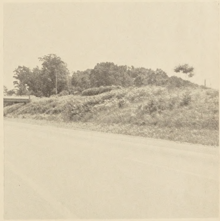
Figure 9.—Slope area left unmowed to encourage regeneration of erosion-proof, natural ground cover.
