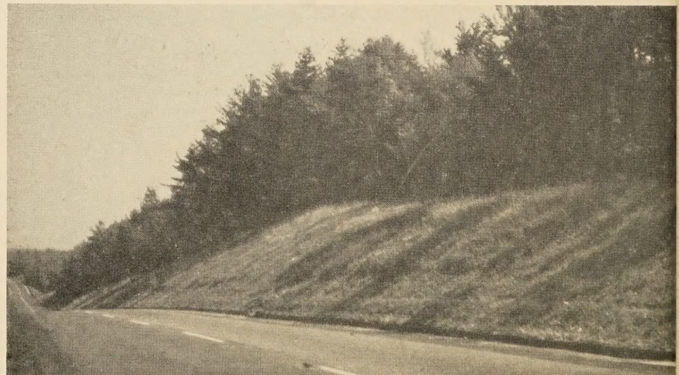
Figure 3.—Slope protected by appropriate ground cover following construction.
