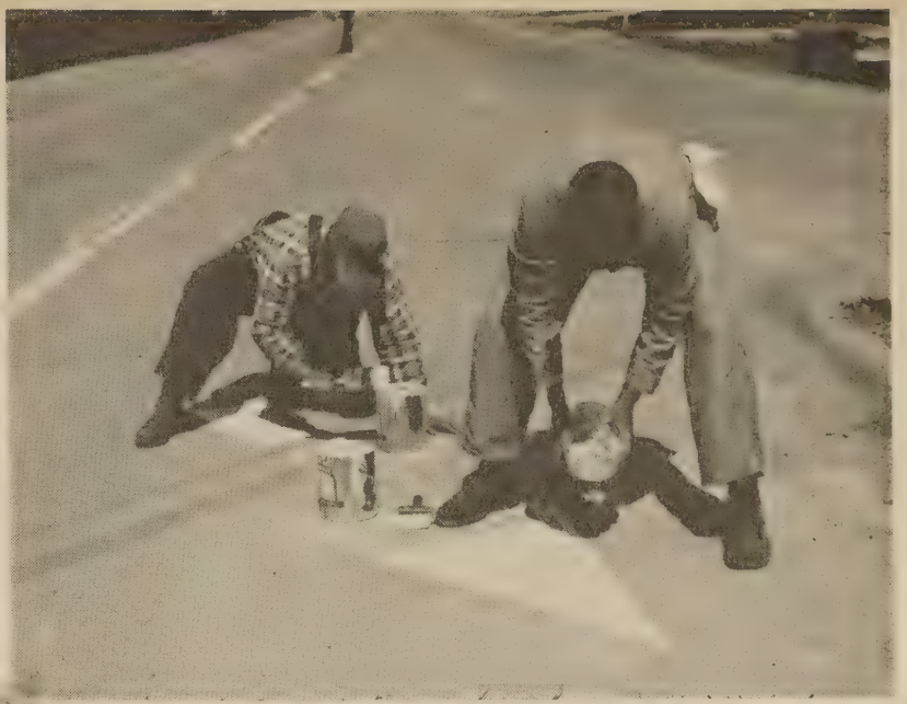
Painting pavement marking
