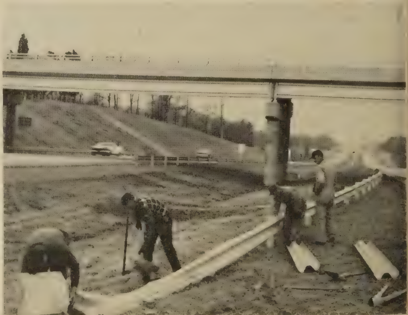
Replacing damaged guardrail
