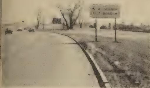
Figure 5.—Dummy sign, black legend on reflectorized white background.
