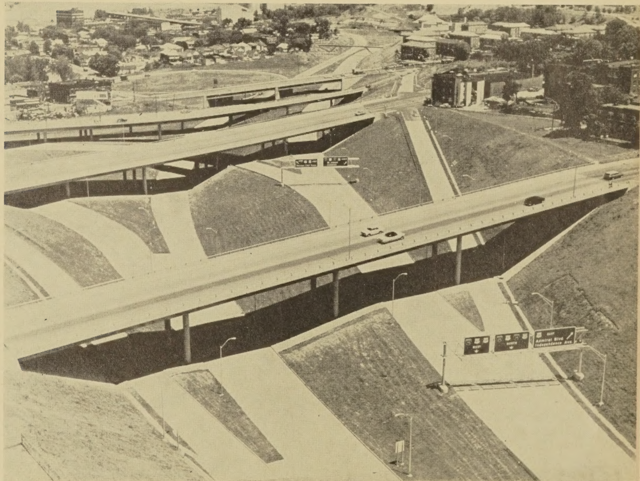
Interchange of Interstate Highways 70, 29, and 35 in Kansas City, Mo.
