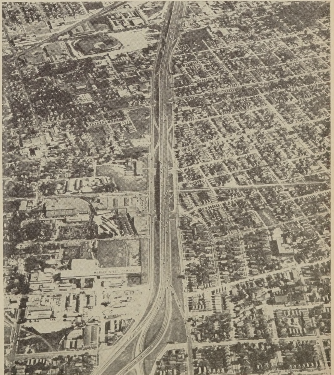
Figure 2.—Varying uses of land near a highway, illustrated by the Gulf Freeway, Houston, Tex.
