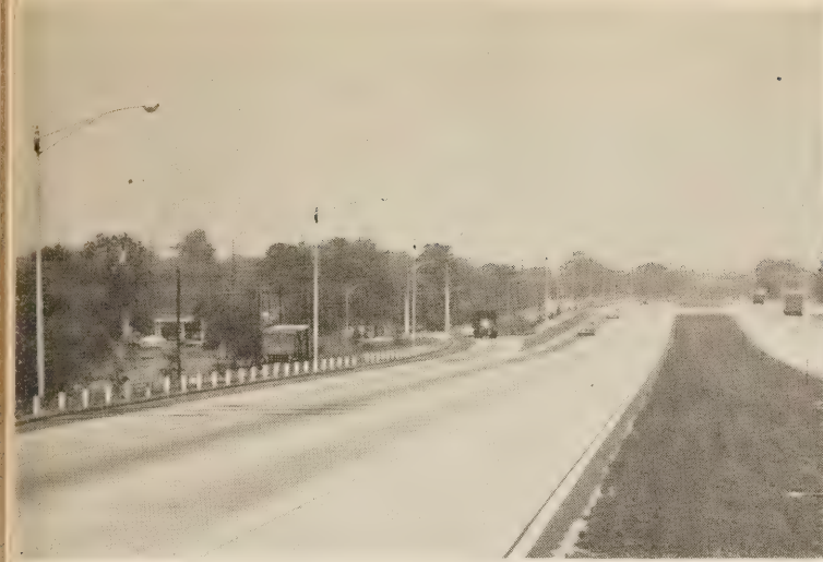
Figure 3.—Access ramp site 4M.
