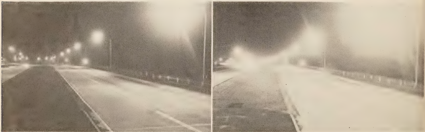
Figure 7.—A section of the Connecticut Turnpike under one-half normal illumination (left) and normal illumination (right).
