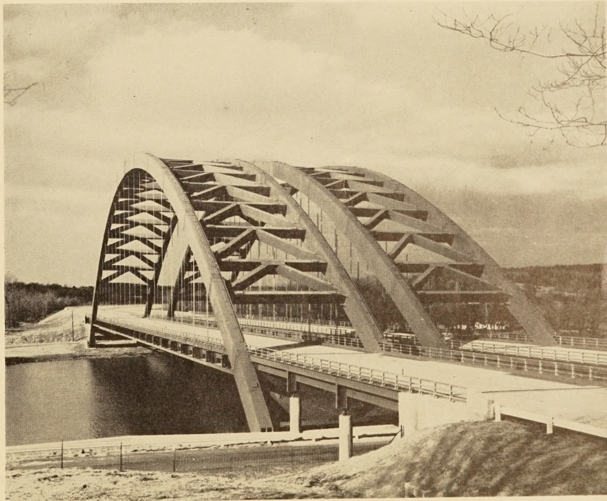
Mohawk River Bridge, Interstate Route 87, near Albany, N.Y.
