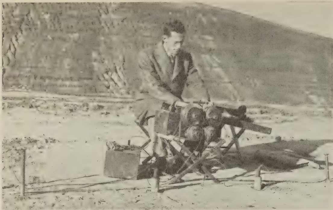
Figure 2.—Earth-resistivity apparatus used by the Bureau of Public Roads in making subsurface explorations.
