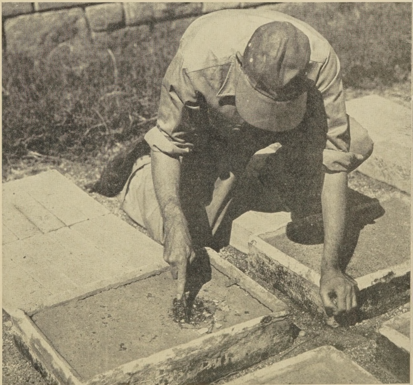
Examining portland cement concrete slabs for scaling action
