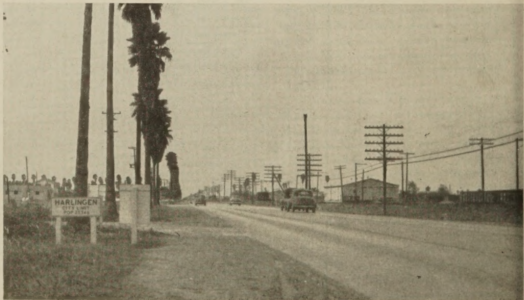
Figure 4.—View of the eastern end of Texas control section 39-6.
