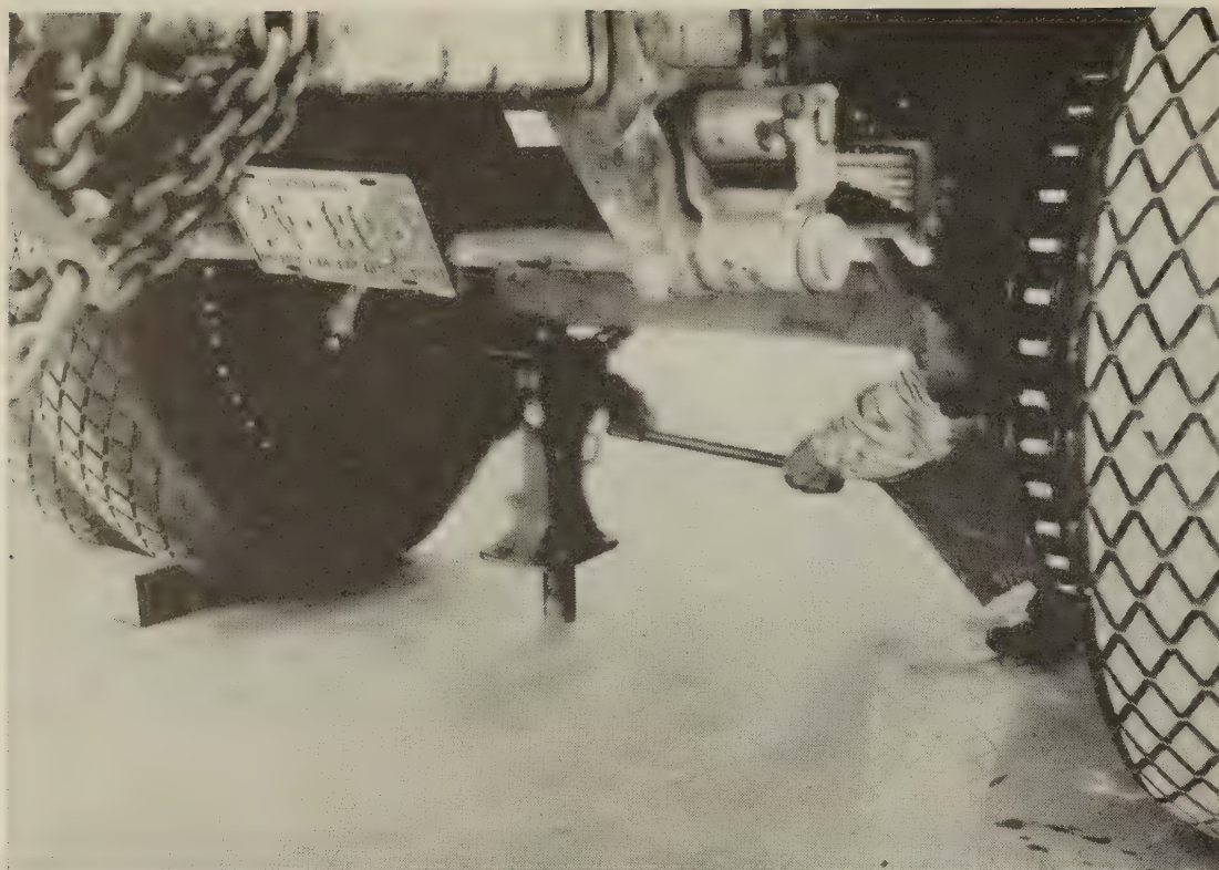
Method of cutting cores for laboratory testing.
