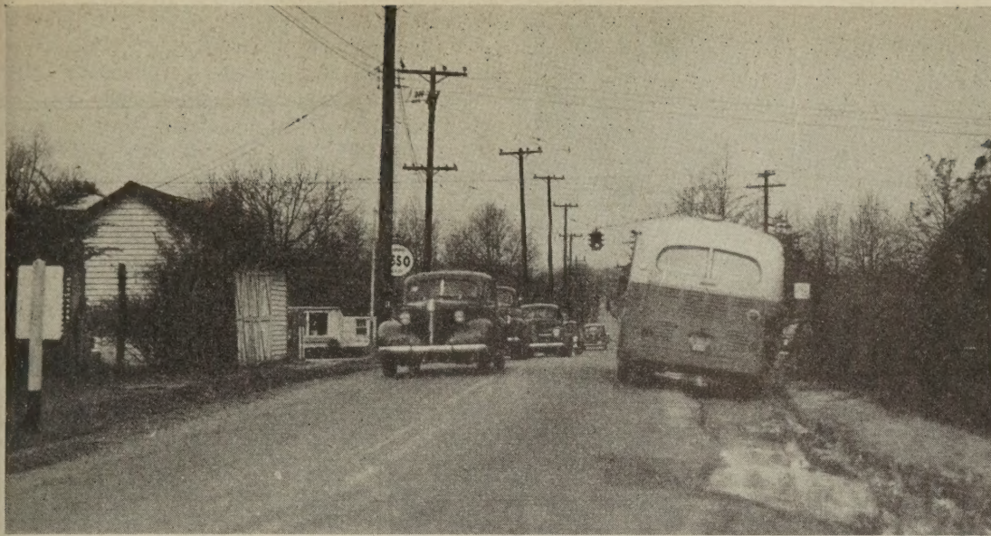
The need for wide shoulders is evident here.
