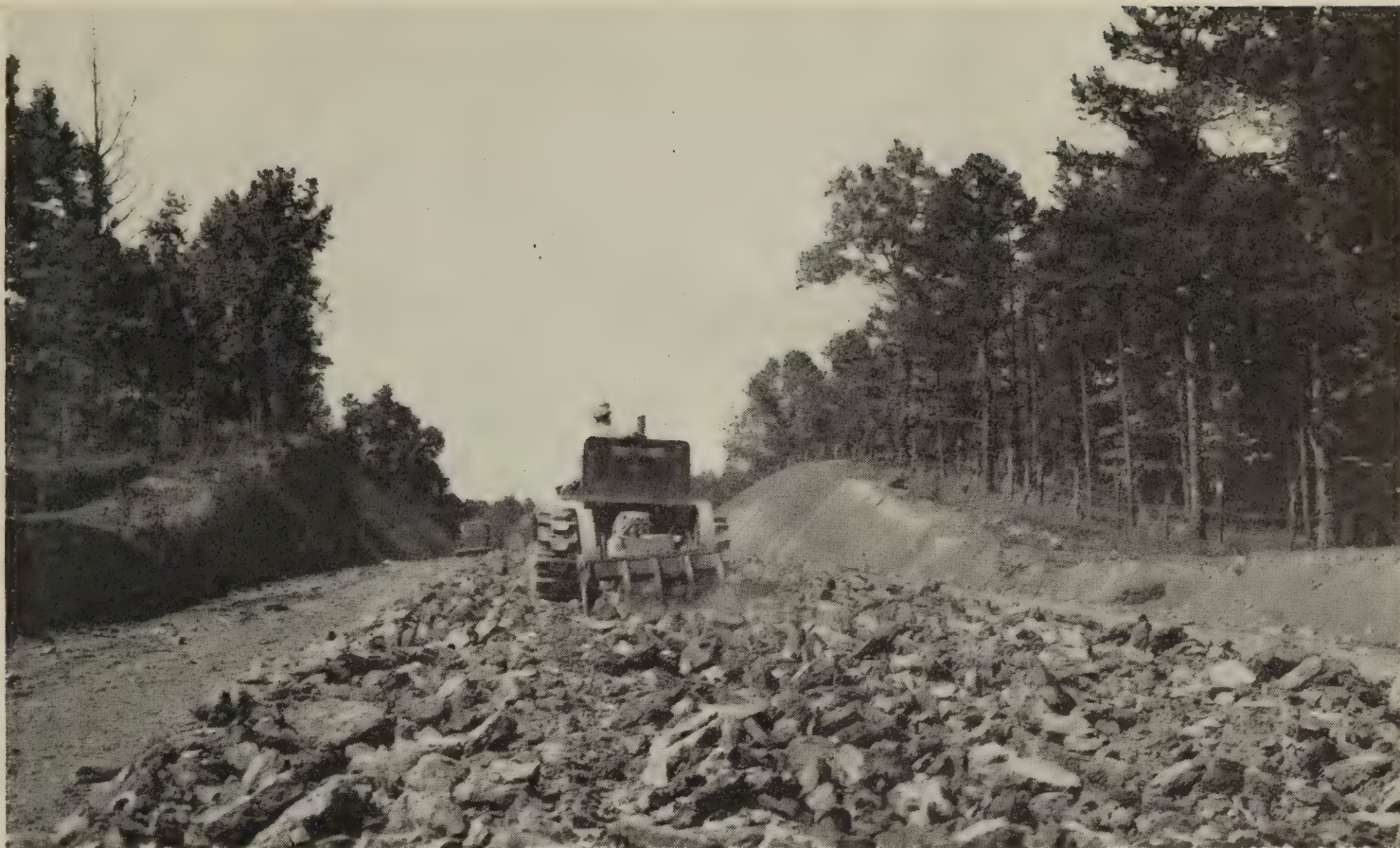
Scarifying hardened soil-cement base course for reconstruction
