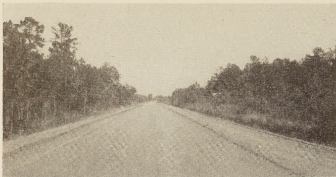
FIGURE 7.—THE COMPACTED STABILIZED BASE PRIOR TO APPLICATION OF BITUMINOUS SURFACING.
