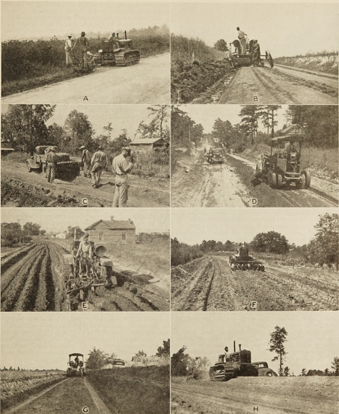
FIGURE 6.—CONSTRUCTION OF SAND-CLAY BASE COURSE: (A) SCARIFYING OLD ROADWAY AND (B) REMOVING MATERIAL TO WIDEN TRENCH SECTION; (C) DISTRIBUTING AND (D) SPREADING NEW MATERIAL FROM BORROW PITS; (E) PLOWING ORIGINAL SURFACE AND ADDED MATERIAL; (F) PULVERIZING WITH DISK HARROW; (G) MIXING ORIGINAL AND ADDED MATERIAL WITH MOTOR GRADER; (H) PULVERIZING WITH DISK HARROW DURING MIXING OPERATION.
