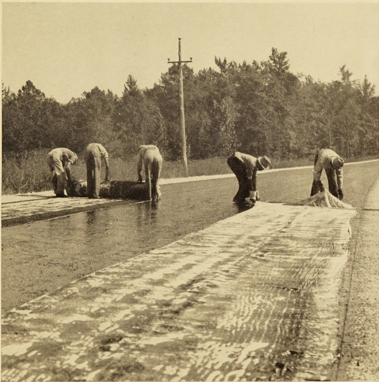
LAYING COTTON FABRIC ON AN EXPERIMENTAL ROAD
