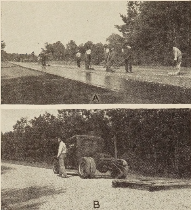
FIGURE 5.—(A) INITIAL HAND-BROOMING INSURED UNIFORM AGGREGATE COVERAGE. (B) A FIBER BROOM DRAG COMPLETED THE SPREADING WHICH WAS FOLLOWED BY MODERATE ROLLING.
