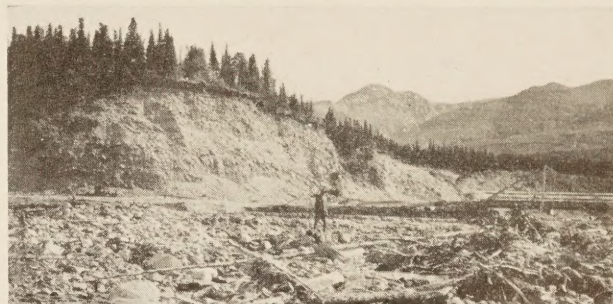
FIGURE 11.—BRIDGE OVER GUNNYSACK CREEK ON RICHARDSON HIGHWAY. AN EARLIER BRIDGE IS BURIED UNDER BOULDERS AT THE POINT WHERE MAN IS STANDING.
