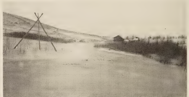
FIGURE 5.—ICE ON STEESE HIGHWAY AT FOX GULCH, MARCH 14, 1933. TELEPHONE WIRES ARE STRUNG ON TRIPODS TO AVOID HEAVING. LITTLE SNOW ACCUMULATED DURING THE WINTER.
