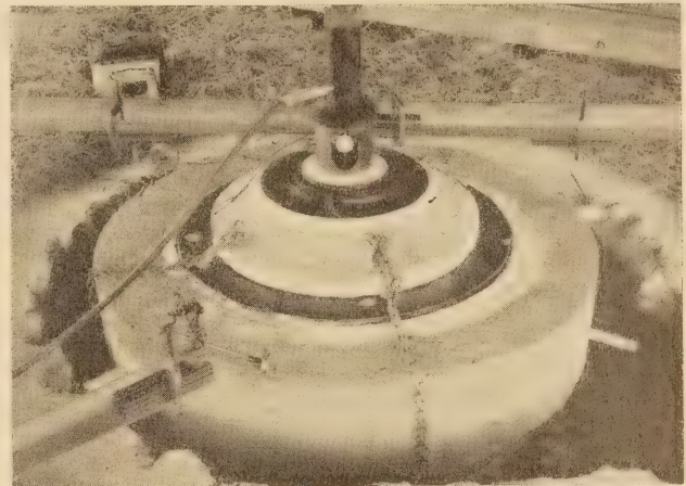
FIGURE 71.—DETERMINING THE MODULUS OF SUBGRADE REACTION WITH A LARGE BEARING PLATE PLACED ON THE SUBGRADE THROUGH AN OPENING CUT IN THE PAVEMENT.
