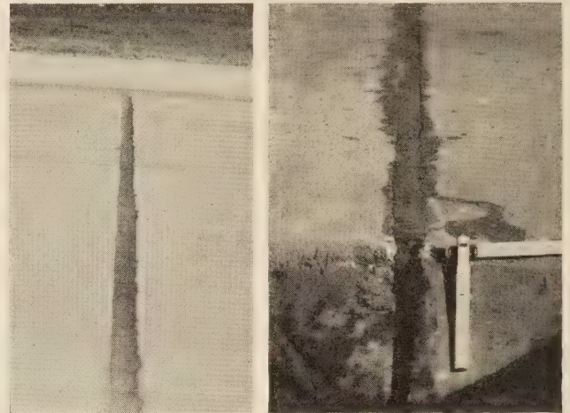
LEFT, A 2-INCH Poured RUBBER COMPOSITION SEAL IN GOOD CONDITION; RIGHT, A Poured RUBBER COMPOSITION SEAL THAT HAS EXTRUDED.
