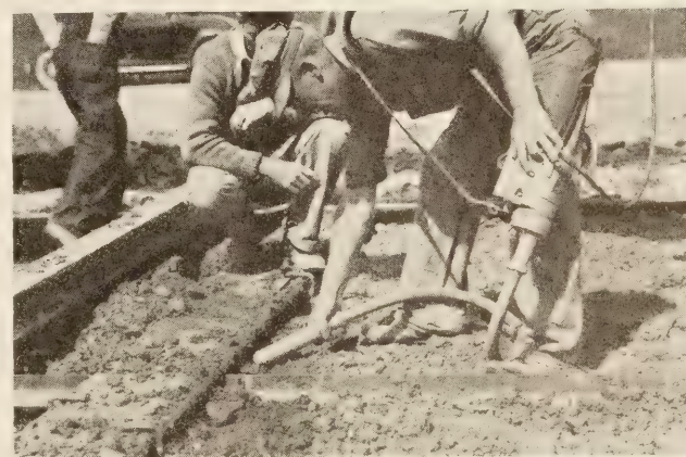
FIGURE 16.—INTERNAL VIBRATOR USED UNDER TYPES I AND II JOINTS.
