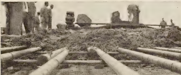
FIGURE 13.—CONCRETE BEING PLACED IN A HEAVILY REINFORCED SECTION.
