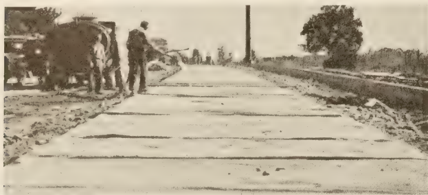
FIGURE 1.—COTTON MATS IN PLACE BEING WET DOWN.
