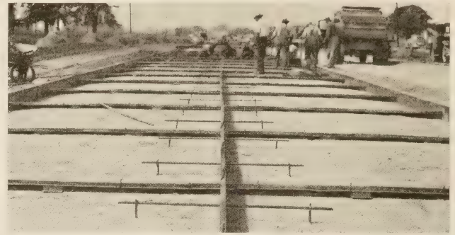
FIGURE 10.—DEVICES USED IN FORMING SUBMERGED WEAKENED-PLANE JOINTS IN PLACE ON THE SUBGRADE.
