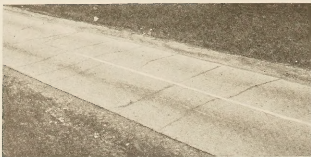
FIGURE 1.—PRESENT APPEARANCE OF A HEAVILY REINFORCED SECTION OF THE COLUMBIA PIKE EXPERIMENTAL PAVEMENT.
