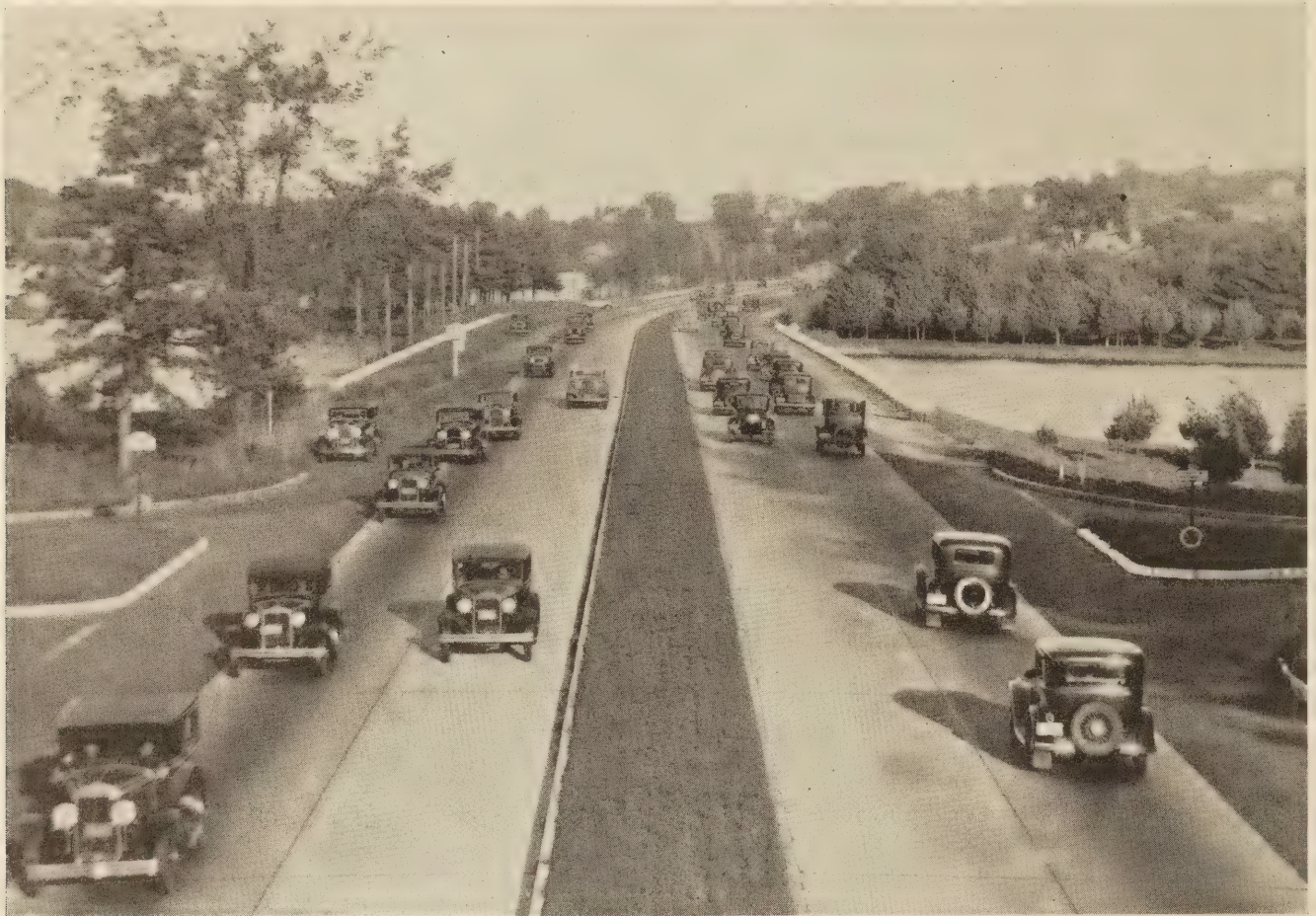
A FOUR-LANE DIVIDED HIGHWAY IN MASSACHUSETTS.
