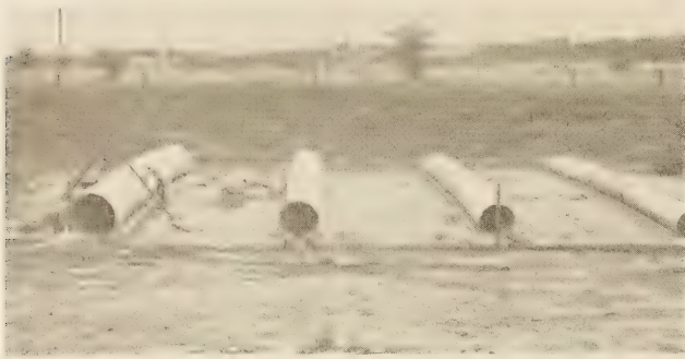
FIGURE 11.—CULVERTS IN PLACE BEFORE THE FILL WAS CONSTRUCTED.
