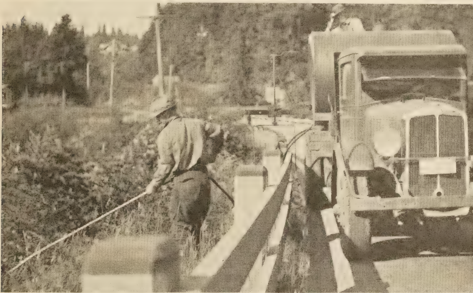
Truck equipped with U-Shaped Device for Spraying Around Posts and Under Rail. Weeds Behind Rail Are Being Sprayed Using a Pipe Attachment.
