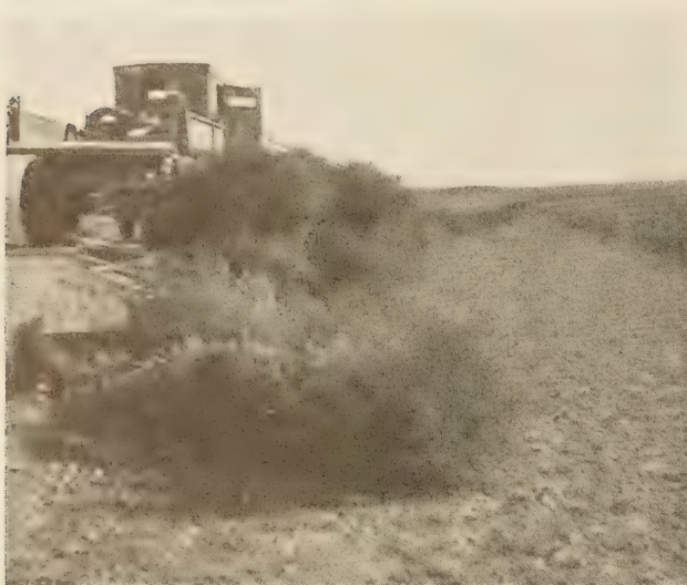
PULLING DRY WEEDS ON A DESERT ROAD BY MEANS OF A WEIGHTED WIRE MESH.
