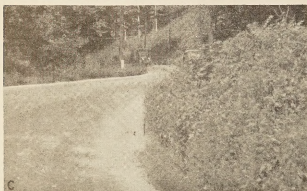
WEEDS MAY BECOME A MENACE TO TRAFFIC: A, BY REDUCING THE EFFECTIVENESS OF GUARDRAIL; B, BY CONCEALING MARKERS AND OBSTRUCTIONS OUTSIDE THE TRAVELED WAY; AND C, BY SHORTENING SIGHT DISTANCES AT CURVES.
