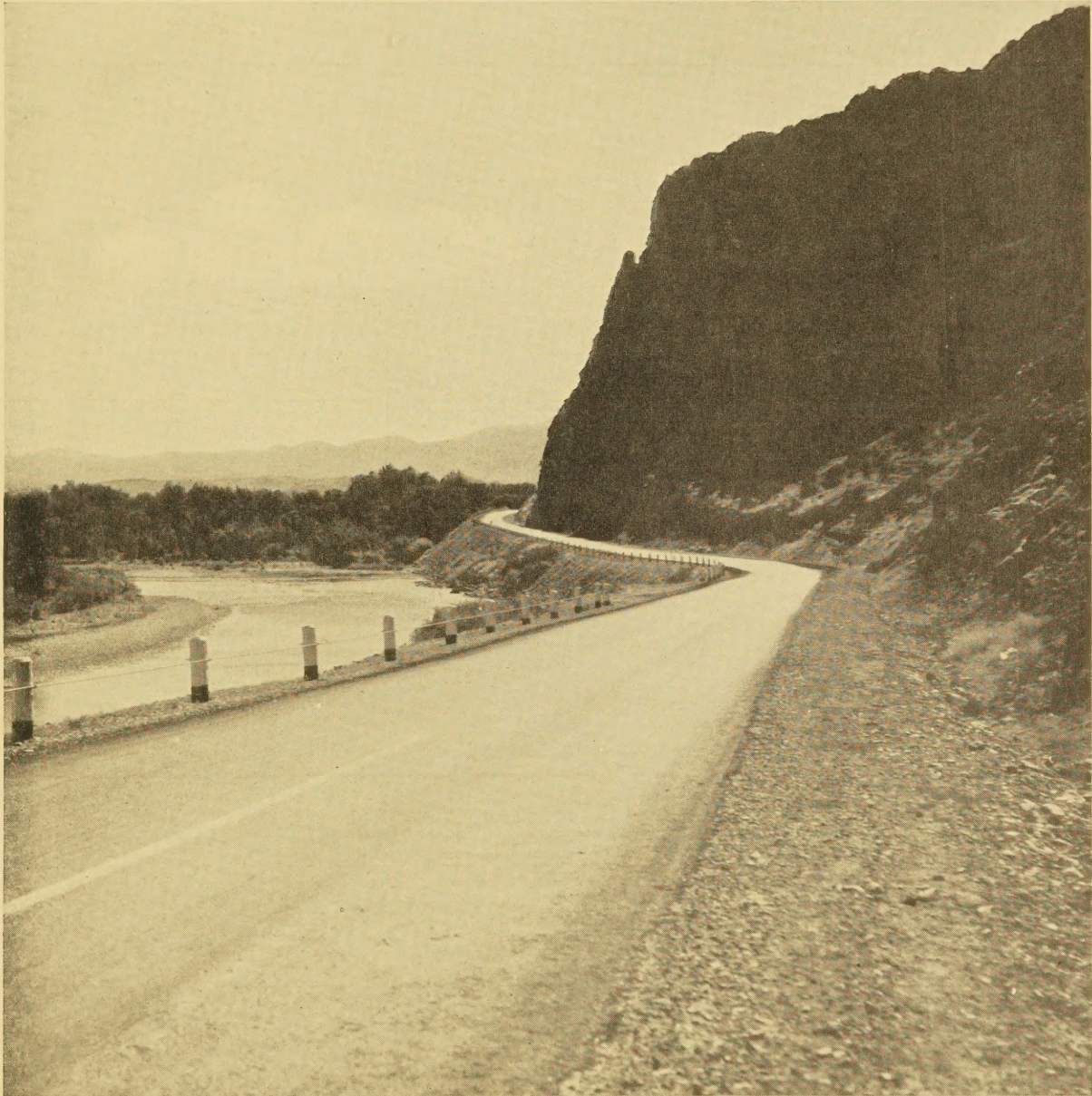
A SECTION OF U S 10 IN MONTANA
