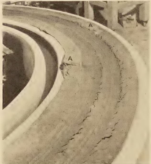
FIGURE 14.—SECTION OF TRACK NO. 10 CONTAINING 5 PERCENT OF MATERIAL C, AFTER 9,000 WHEEL TRIPS OF DISTRIBUTED TRAFFIC AND 500 WHEEL TRIPS OF CONCENTRATED TRAFFIC. MUD WAS EJECTED FROM THE SPOTS MARKED "A".
