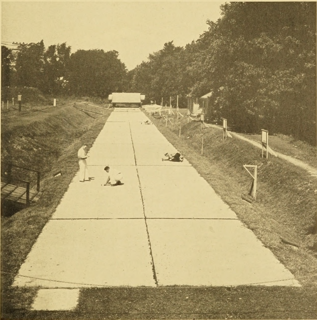
FULL-SIZE PAVEMENT SLABS TESTED AT ARLINGTON EXPERIMENT FARM
