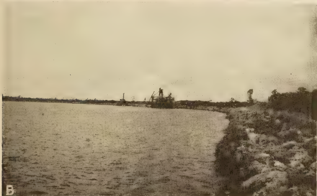
FIGURE 2.—METHODS OF MINING LIMEROCKS: A, OPEN-PIT MINING OF OCALA LIMEROCK; B, DREDGING OF MIAMI OOLITE.
