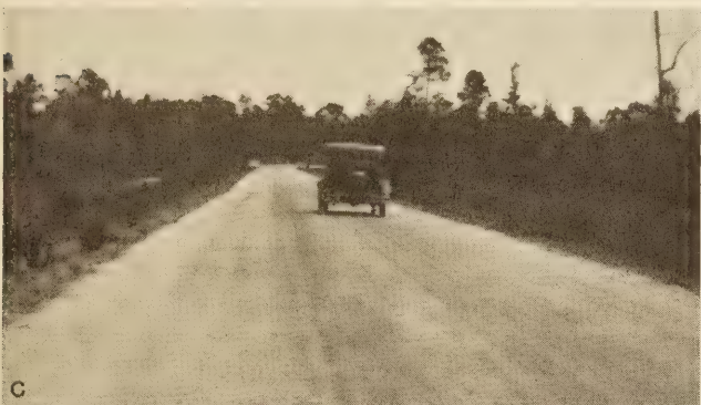
FIGURE 4.—A, COMPLETED LIMEROCK BASE COURSE WITH PRIME COAT; B, APPLYING SURFACE TREATMENT; C, SURFACE TREATMENT COMPLETED AND HIGHWAY IN USE.
