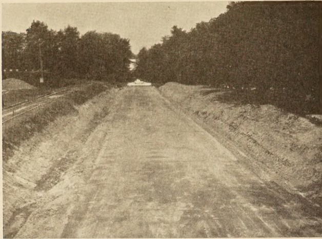
FIGURE 4.—APPEARANCE OF THE SUBGRADE AFTER ROLLING HAD BEEN COMPLETED.
