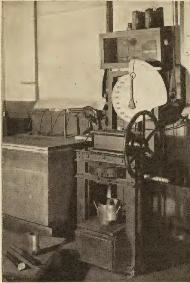
FIGURE 1.—HUBBARD-FIELD STABILITY TESTING MACHINE.
