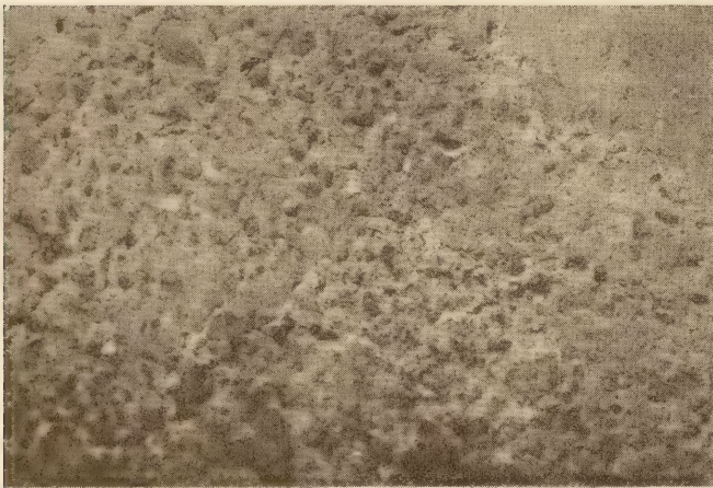
A.—MOTTLED SLAB. SERVICEABILITY NOT REDUCED. AGE 7 YEARS
