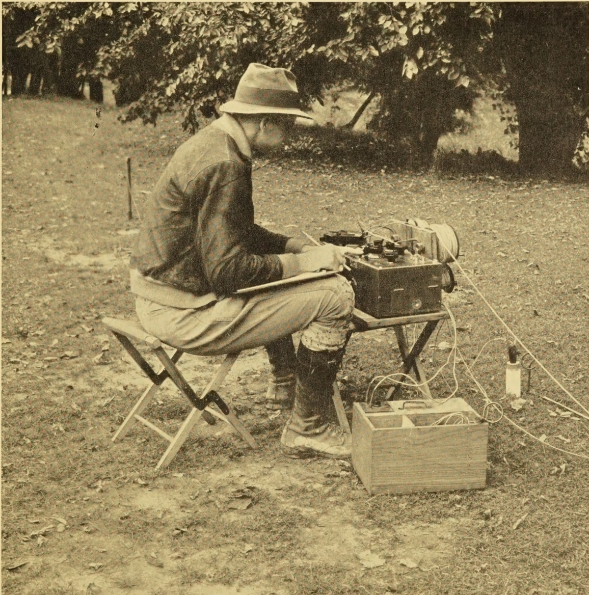
DETERMINING DEPTH TO ROCK BY MEASURING EARTH RESISTIVITY
