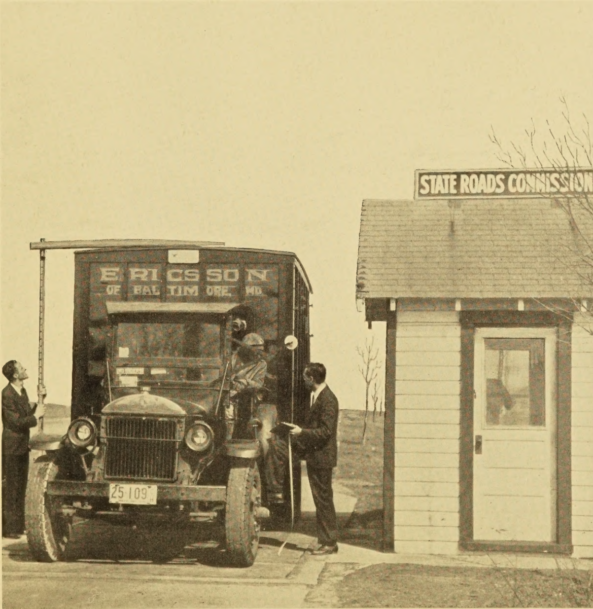
ROADSIDE STATION FOR DETERMINING WEIGHTS AND DIMENSIONS OF TRUCKS
